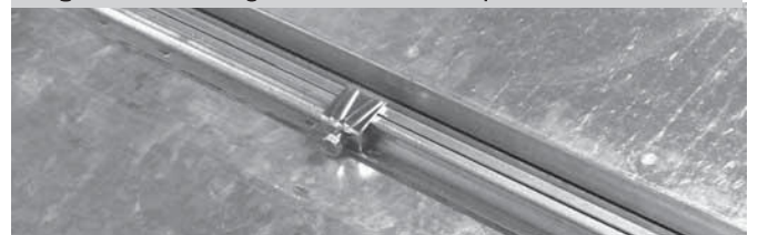
Figure 13 - Flange bar screw clamps
