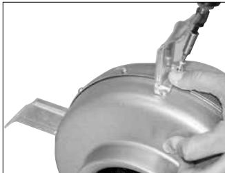
3. Fasten the mounting brackets with the self-drilling screws.
