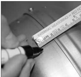
2. Mark the measure of **C**. Start from the joint of the fan.
