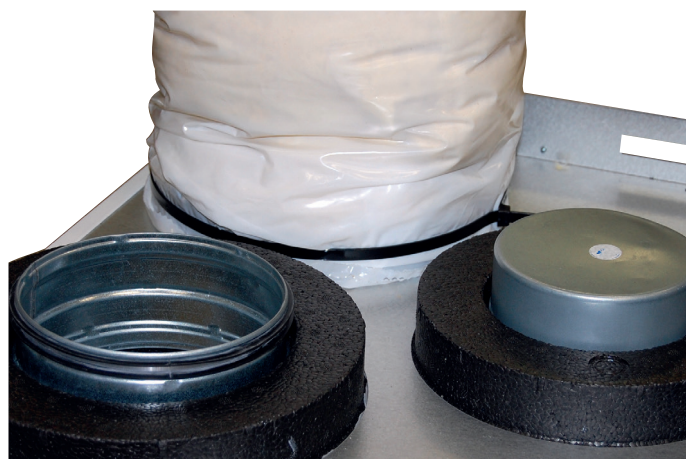
Figure 21 Fitted duct.
