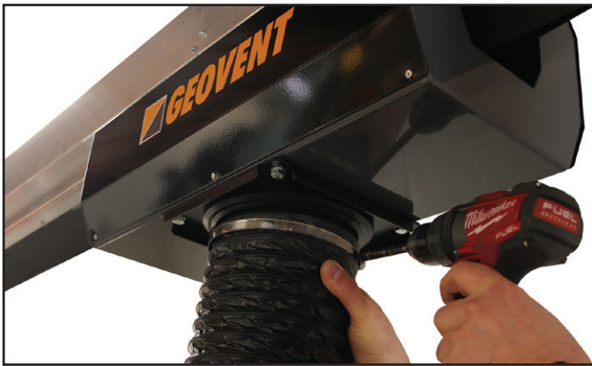
Pull the hose and clamp on to the flange and tighten it.
