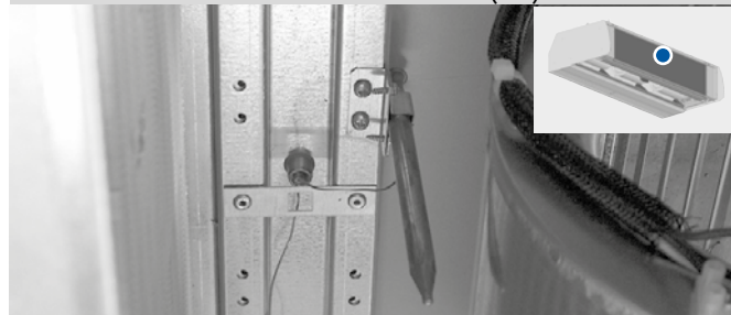
Illustration 17 - thermo-valve's feeler (D2)
