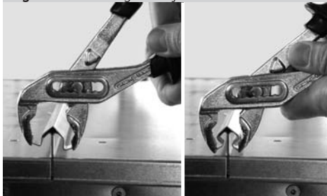
Figure 11 – Covering of roof joints
