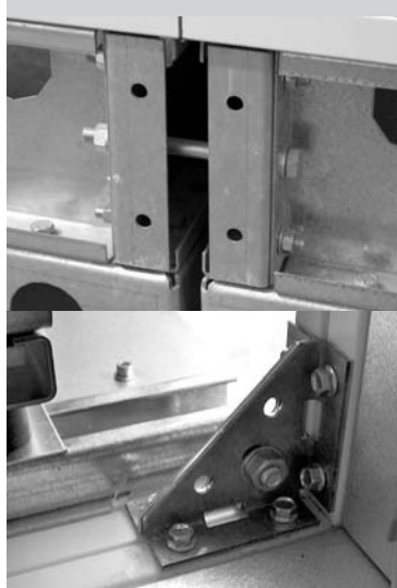
Figure 9 – Connection of frames and connection of sections using corner irons
