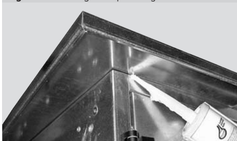
Figure 13 – Sealing of the panel edges
