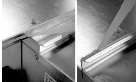
Figure 10 – Sealing of roof elements
