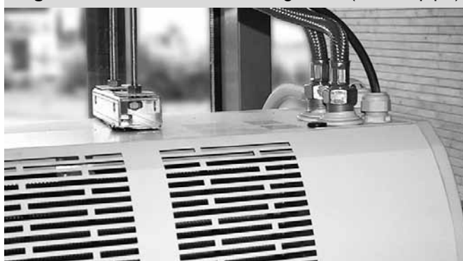
Figure 13 - connection of heating water (flexible pipe)
