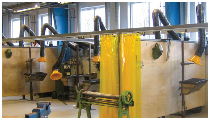
Wing arms \varnothing 160\text{mm} 3m installed at technical school. Including automatic control devices for automatic start/stop of fan and motor damper.
