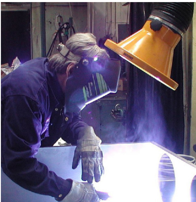
Compact arm 1-2m installed and including automatic control devices for automatic start/stop of the fan and motor damper.
