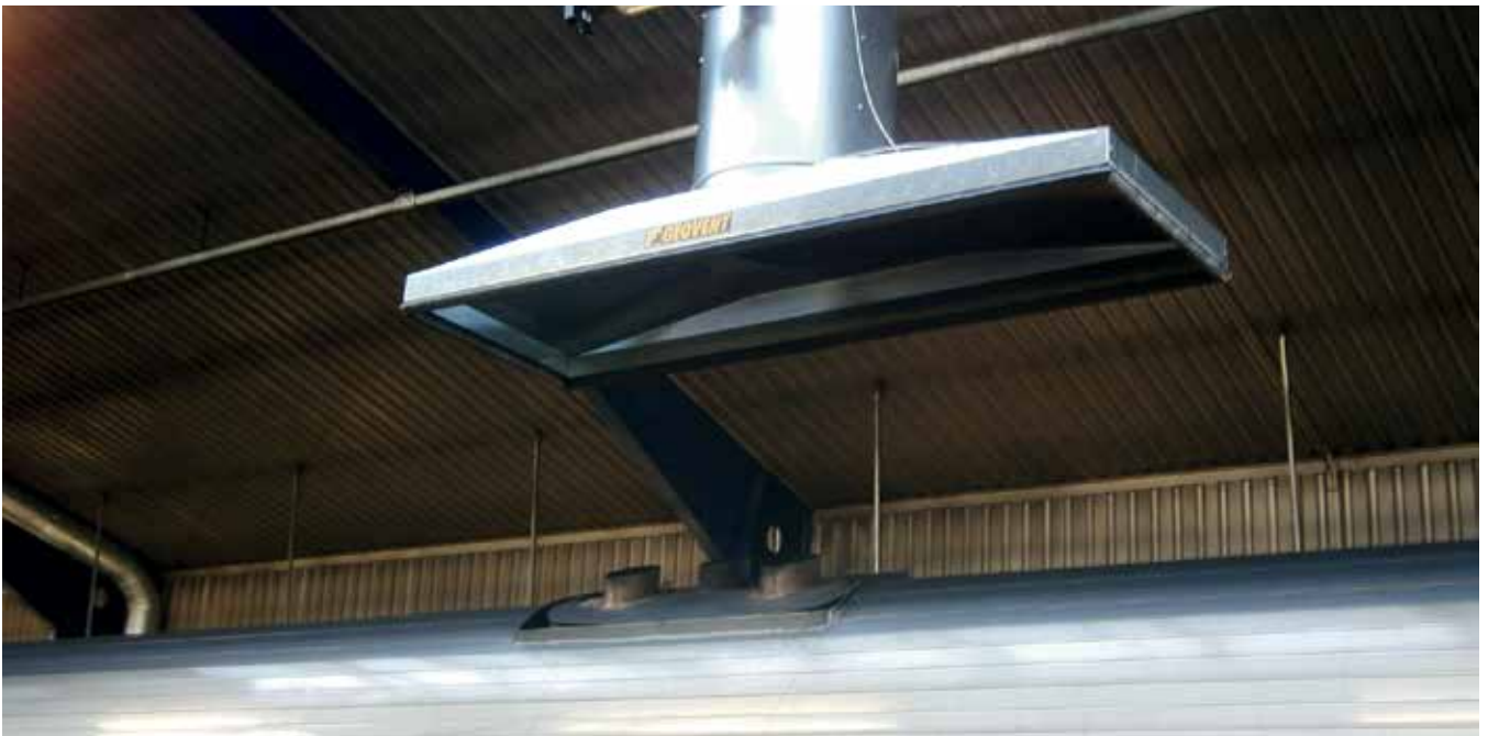
Extraction Hood for train
