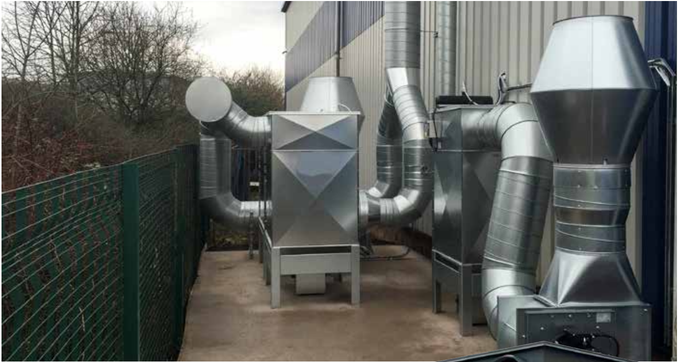
Project with 2 complete filter systems and pressure controlled fans.
