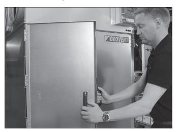
2. The door opens (the filter can be replaced)
